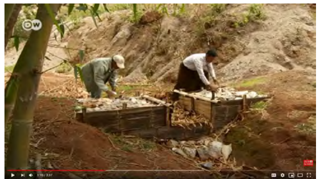
Building terraces to slow down erosion and keep sediment out of the river that is killing fish Screenshot from “Soil Erosion Round the World – Causes and Solutions” from DW News: youtu.be/s0F2c1ECuo4
