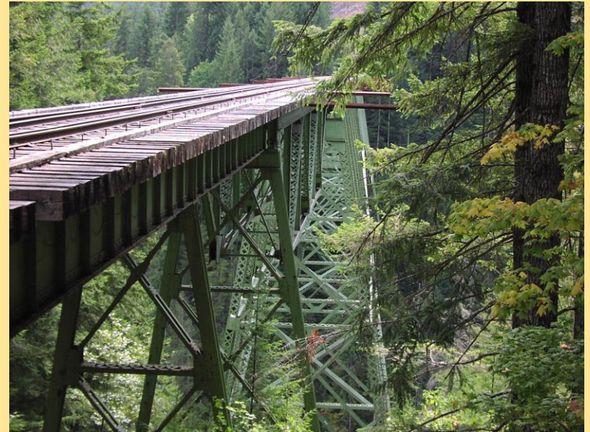
The steel bridge at Gridsale over Vance Creek looking north
