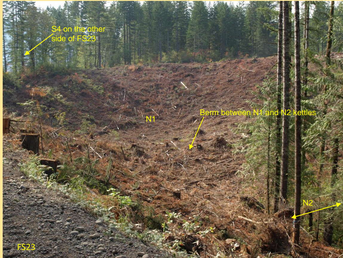
Kettles N1 and N2 next to FS23 at milepost 1.7
