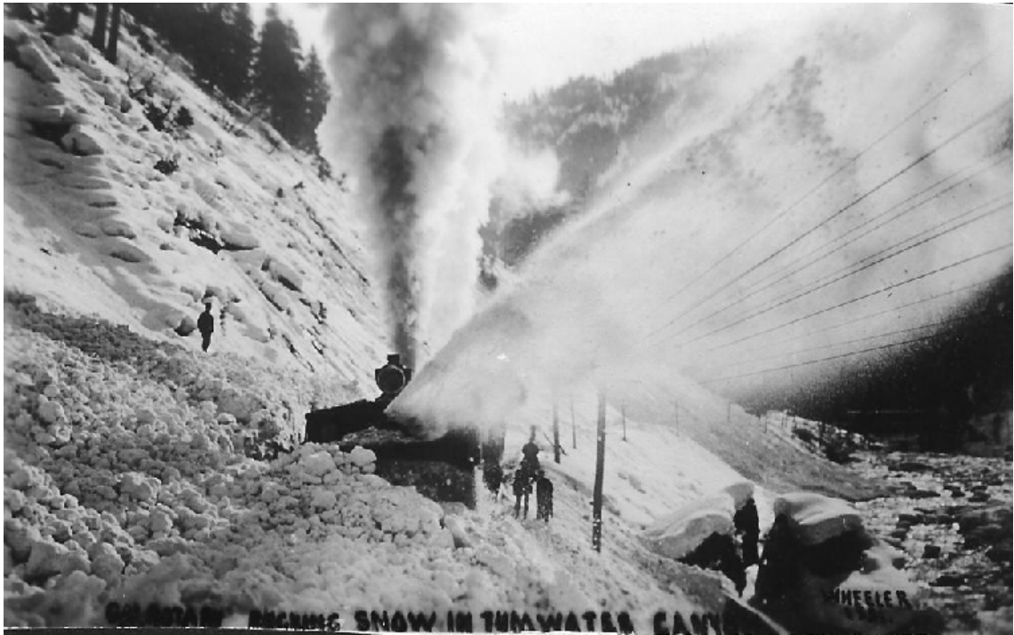
Figure 14. Rotary plow clearing snow from Great Northern tracks in Tumwater Canyon, ca. 1917. Powerlines visible are from generating plant on river side of railbed. View downriver. Source: Ray Wheeler photo, Washington State Historical Society.
