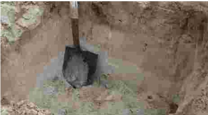
**Figure 1.** Mount Mazama ash encountered in excavation for concrete footings.
